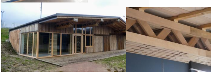
Beech wood construction with pinned joints (Vélo's house, Xertigny, 88)
