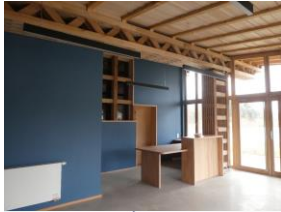
Beech wood construction with pinned joints (Vélo's house, Xertigny, 88)
